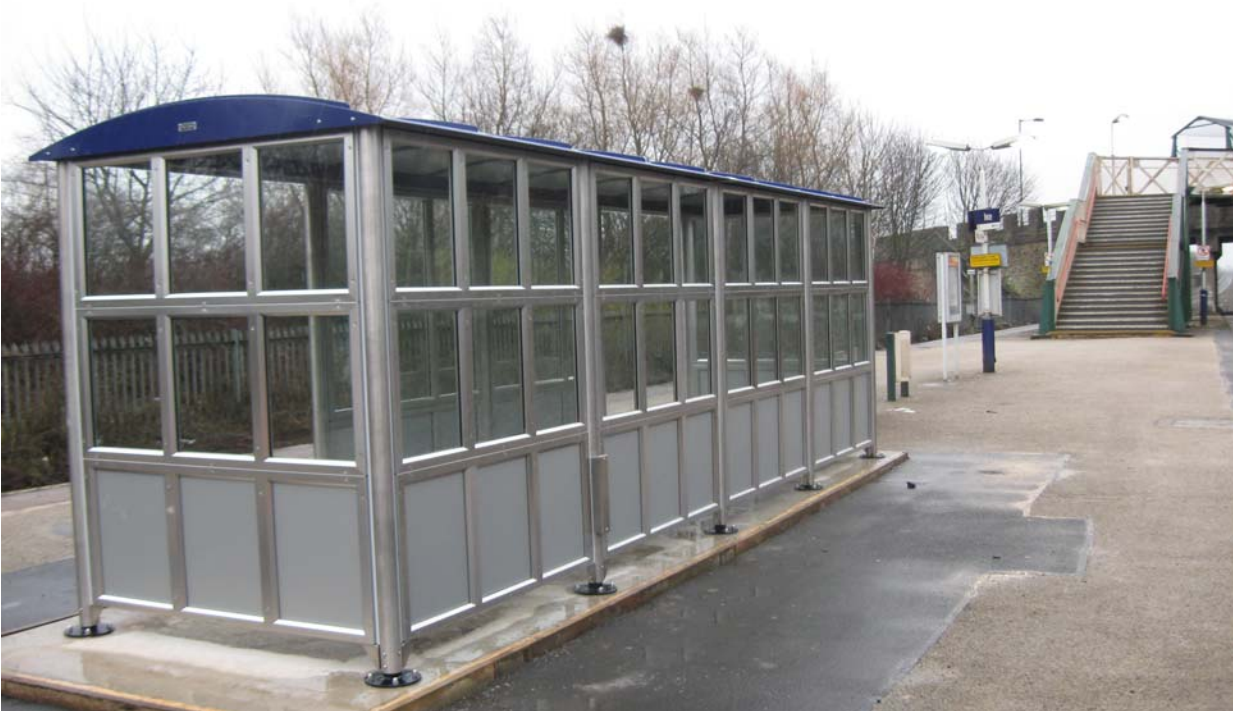
New shelter at Ince.
